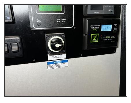
Turn the solar disconnect knob to the "ON" position on the control panel.
